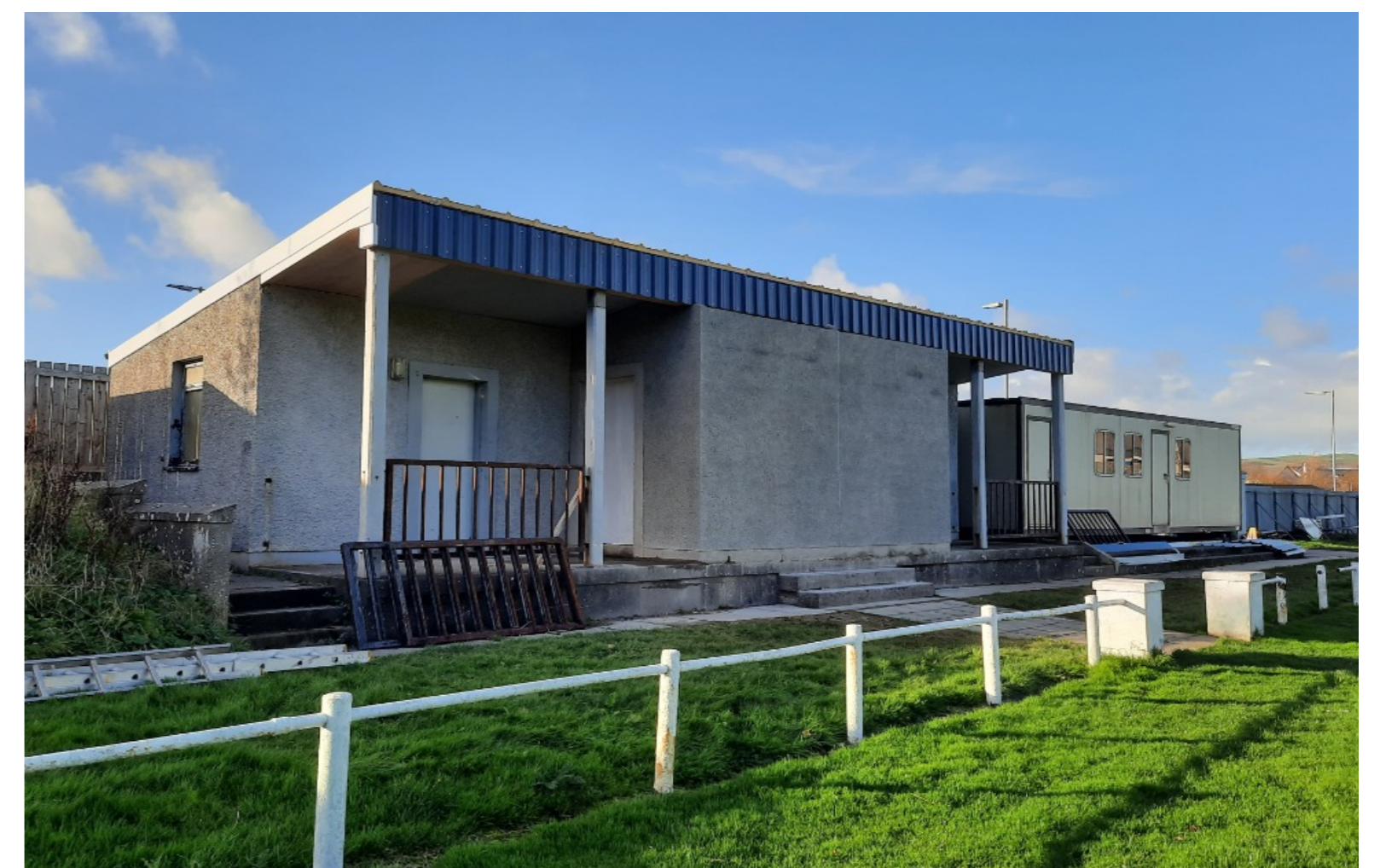
The new match officials extension at Kintyre Park
