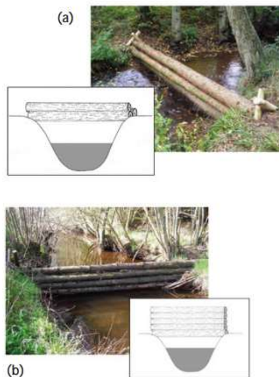
Plate 16 - Examples of different types of in stream placements with low and high vertical height and schematic inset. © Nisbett et al. 2015 [within Dodd et al. 2016]
