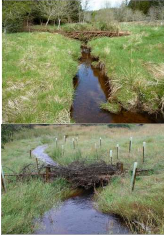
Plate 15 - Leaky dams/ large woody debris in the Eddleston catchment, Scottish Borders. Credit: Tweed Forum
