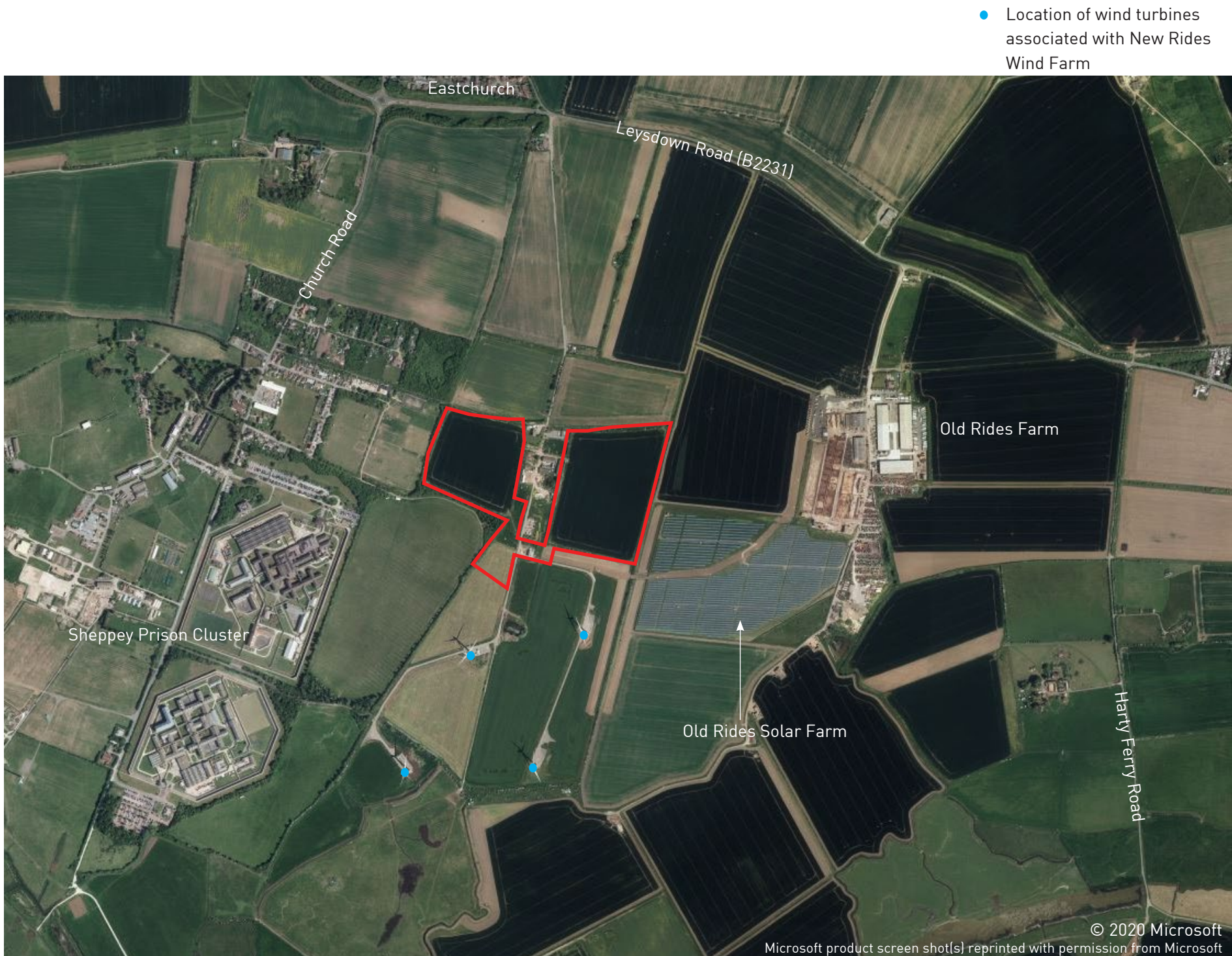
Figure 8: Aerial Photograph of site and surroundings
