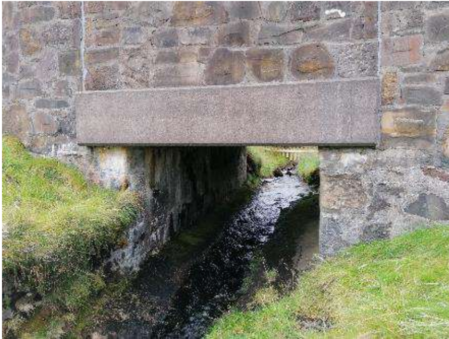
Plate 1: TN 6 Road bridge across Ferly Burn, otter scat underneath.
